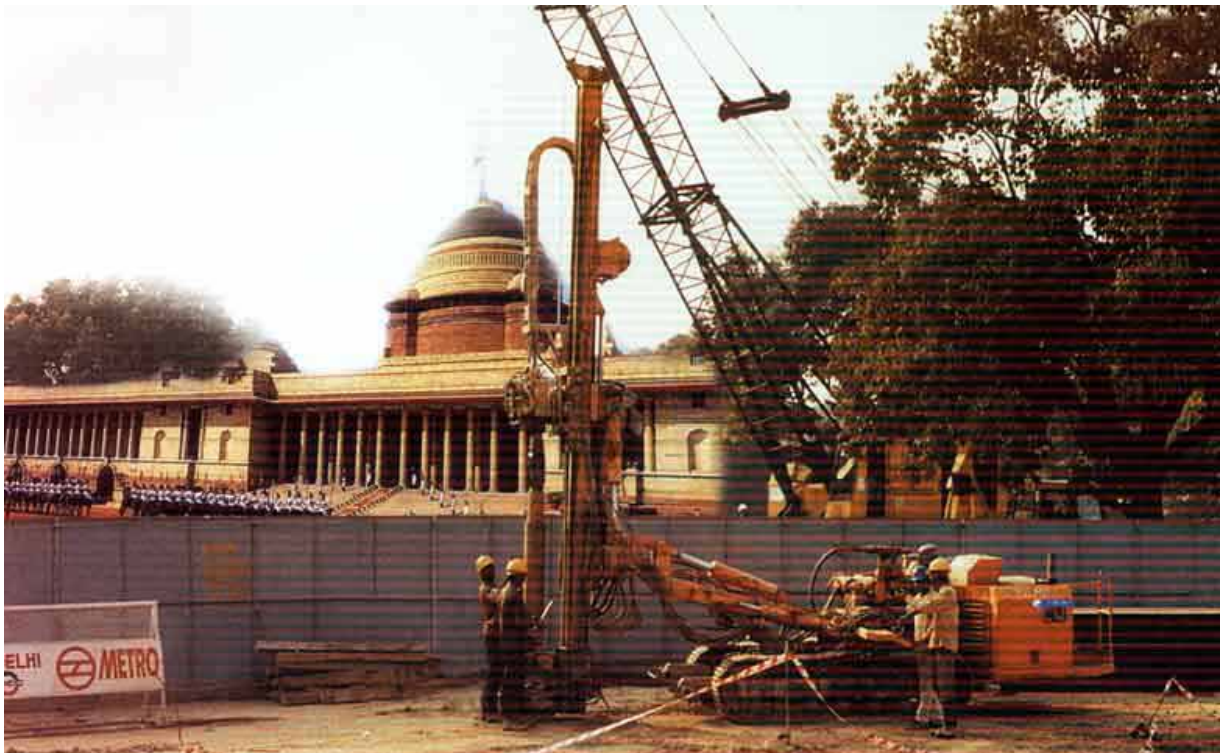
Tubular Kingpost at CS station MC1B, Delhi Metro Rail Corporation, New Delhi, India
