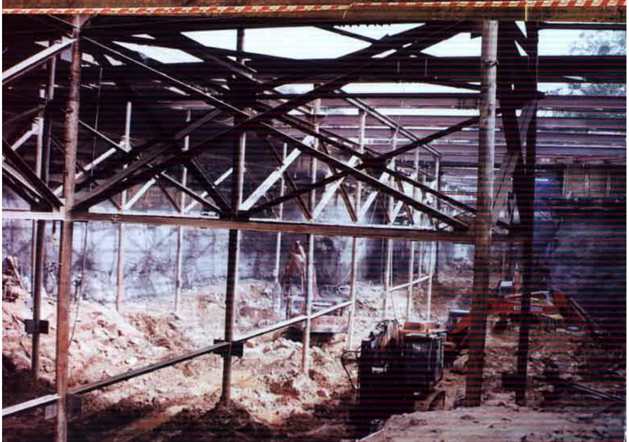
Tubular Kingpost at CS station MC1B, Delhi Metro Rail Corporation, New Delhi, India
