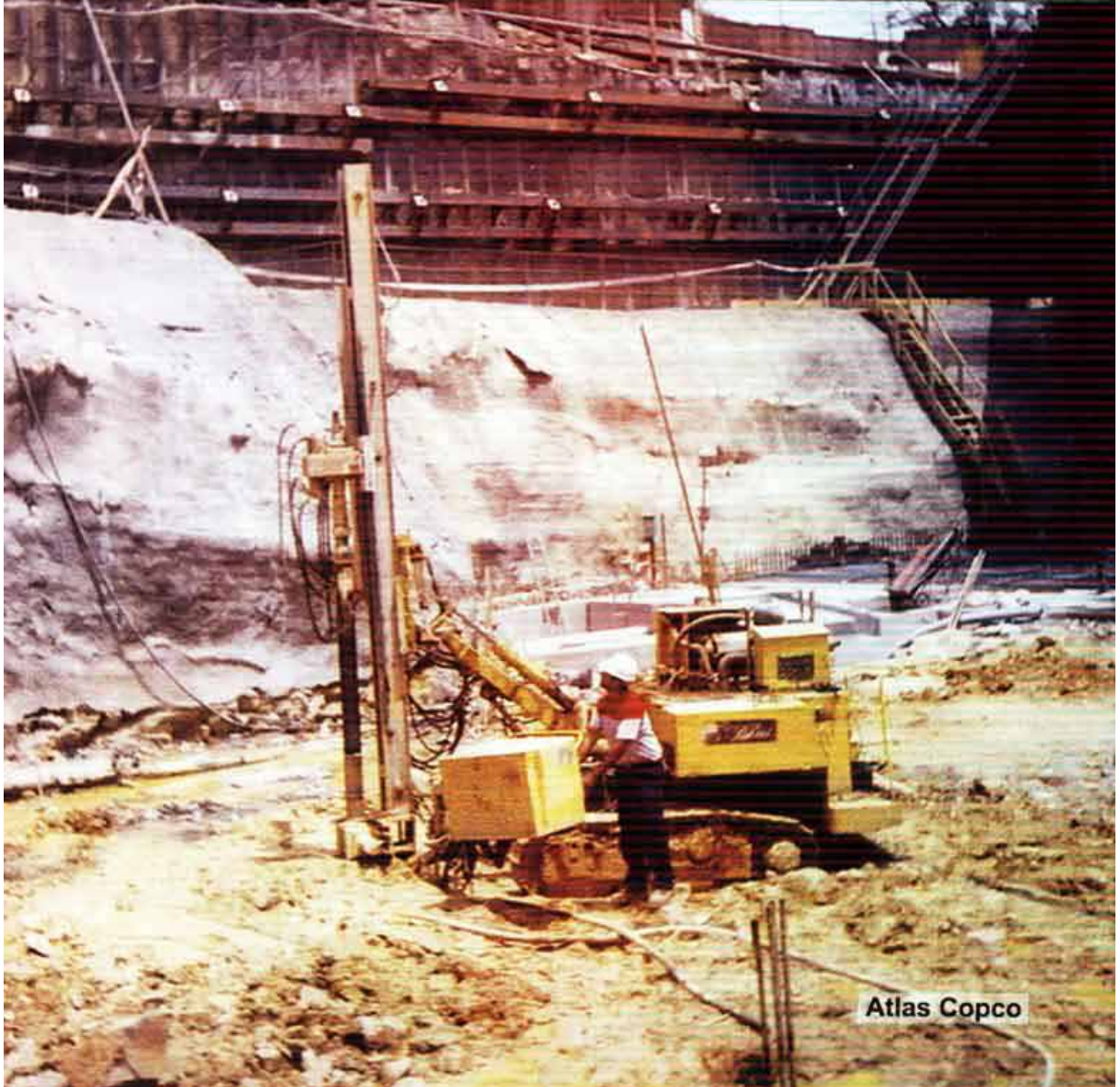
Bauer Anchor hole Drilling Rig with Top head hammer
